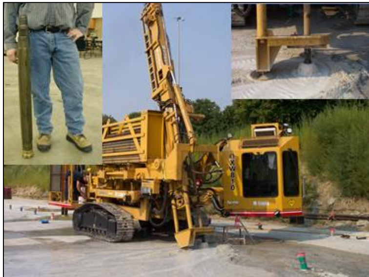
Figure 3. Photo of rotary percussion drill with water activated Down-the-Hole Hammer (Upper Left).
